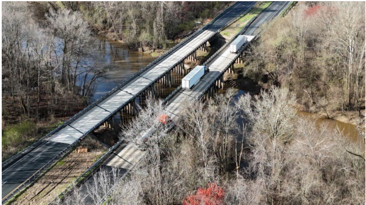
FIGURE 8. NEUSE RIVER BRIDGE
