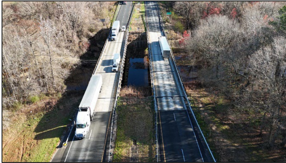
FIGURE 2. BRIDGE NOS 000000001010082 AND 000000001010085 OVER BLACK CREEK
