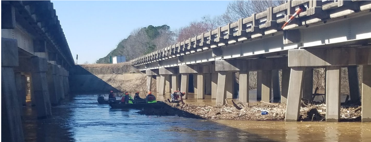
FIGURE 5. DEBRIS REMOVAL AT THE I-95 BRIDGES OVER THE NEUSE RIVER
